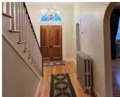
The new wood floor matches the uncovered and refinished floors in the Crown Jewels Gallery and the Peoples Room. The mahogany paneled double door is modeled after historic photos, and an antique chandelier welcomes you.
