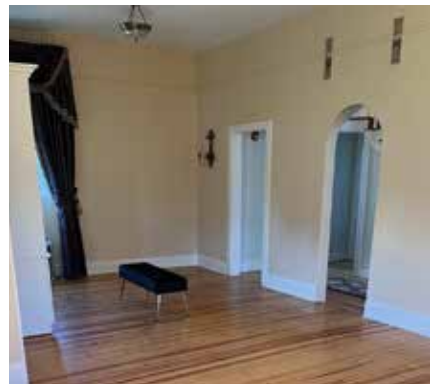
Crown Jewels Gallery work completed.
